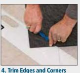
Cut angled corners during installation and trim during use to reduce potential lifting.
