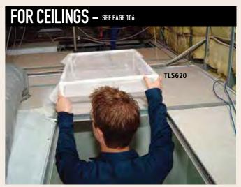
PIG Ceiling Tile Leak Diverters install in office areas for low-profile protection that won't get in your way.
