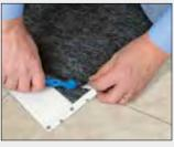
Trimming Edges and Corners If edges become worn or begin to lift, peel back mat until fresh adhesive is exposed, trim and press the new edge into place.
